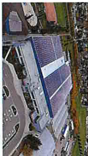
Camrose Rec Centre Solar Array
